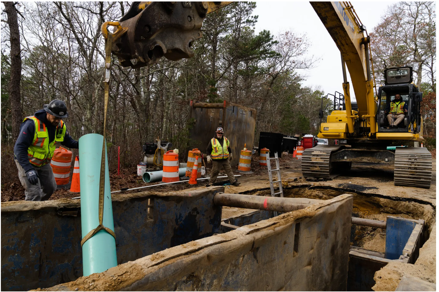
Workers installing a sewer line in Mashpee.
